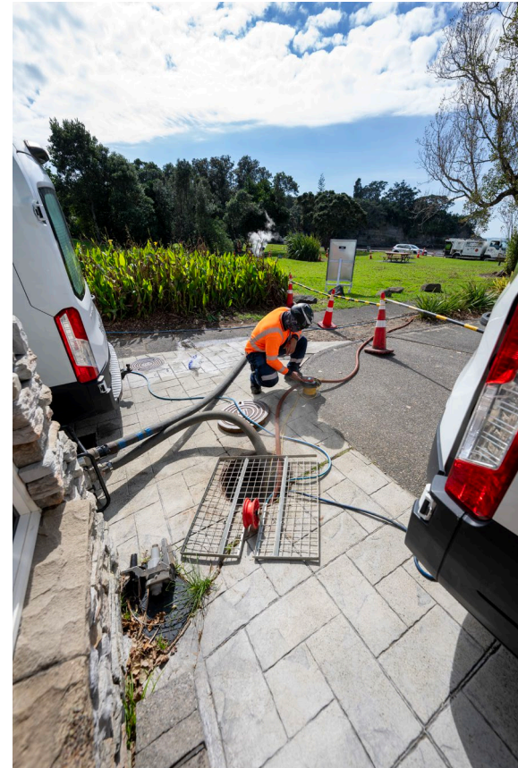
Wastewater renewals underway at Castor Bay.
