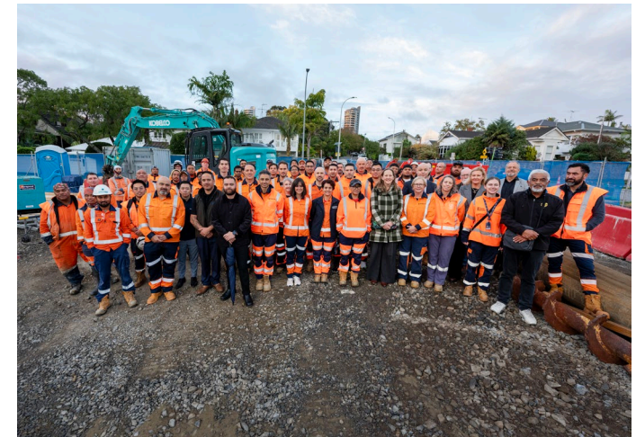
Crews gather for dawn blessing for Herne Bay Collector project.
