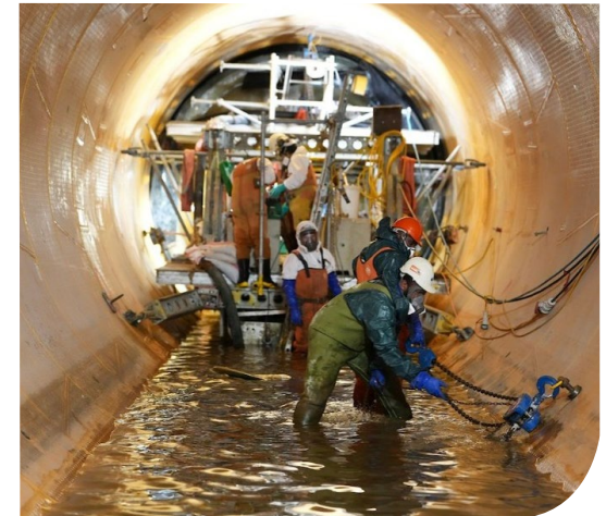
The removal of the bulkhead separating the northern and southern sections of the Central Interceptor reconnected the tunnel for the first time since construction began.
