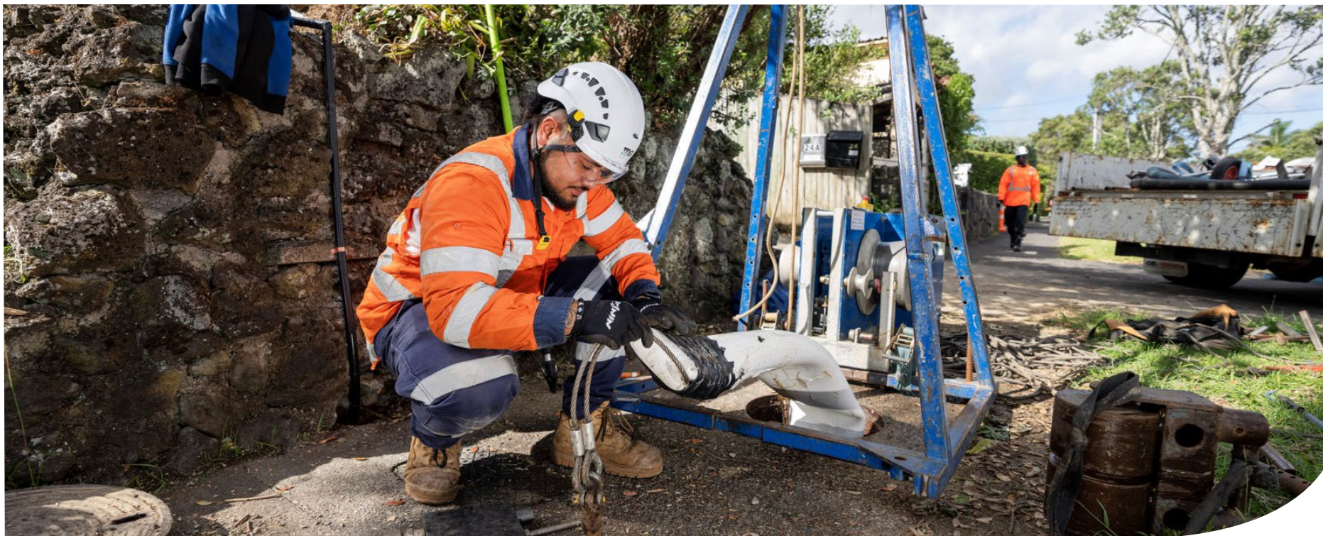
Wastewater renewals underway at Waterview.
