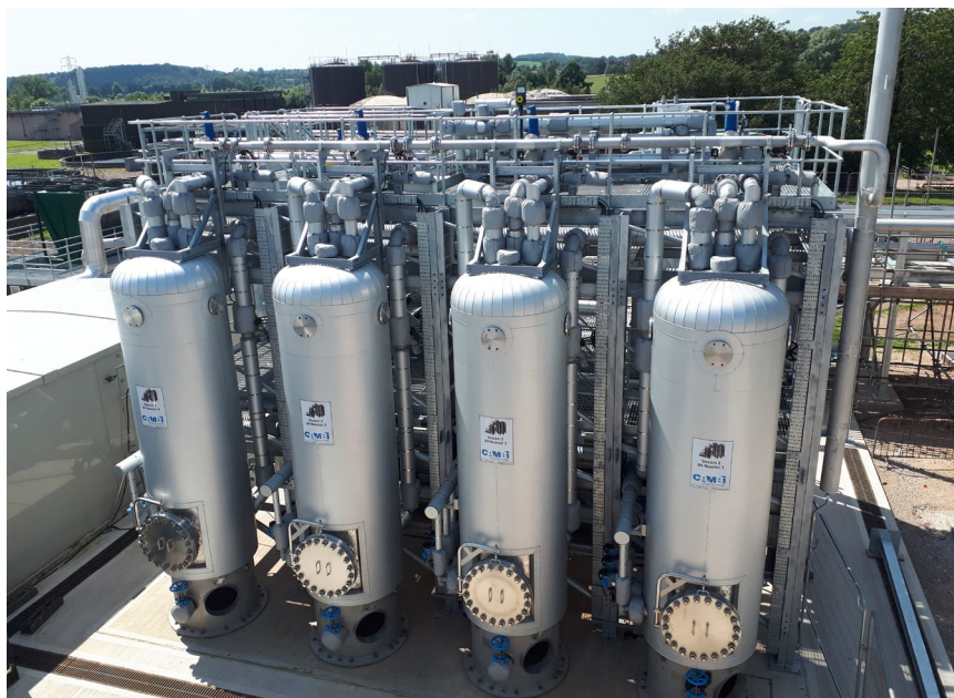
Left: An example of thermal hydrolysis process systems. Photo credit: Cambi
