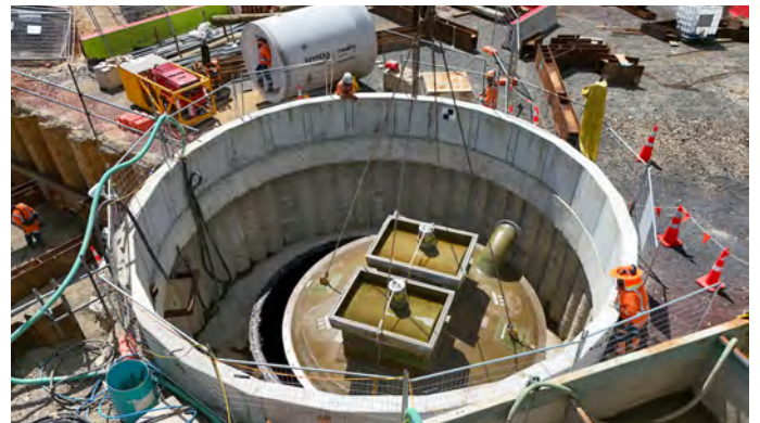
GRP lid being moved into place
