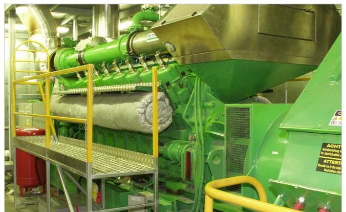
One of the four Jenbacher JMS 616 turbo-charged gas engine/generators.
