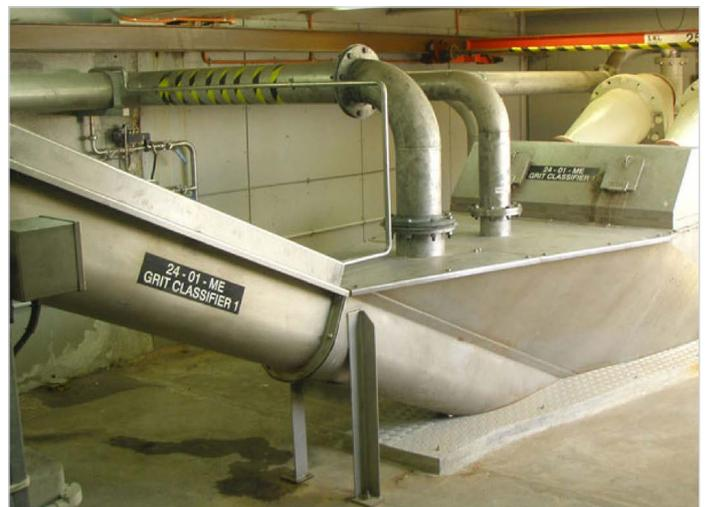
Incoming screened sewage is sent to one of 12 grit removal tanks which are at the head of each primary sedimentation tank.
