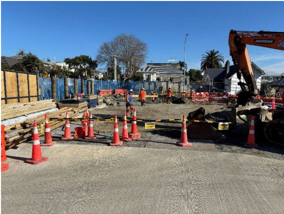
Figure 3 – Looking west towards proposed location of MH02
