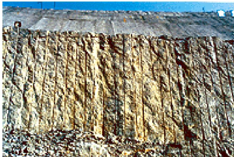
**Figure 1: Example of controlled blasting rock face.**
