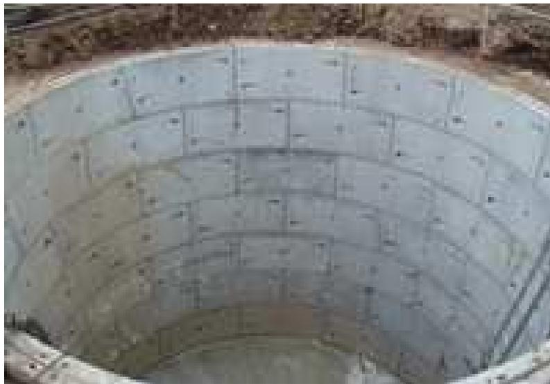
**Figure 2: Example of segmental lining for shaft sinking (perco.co.uk).**
