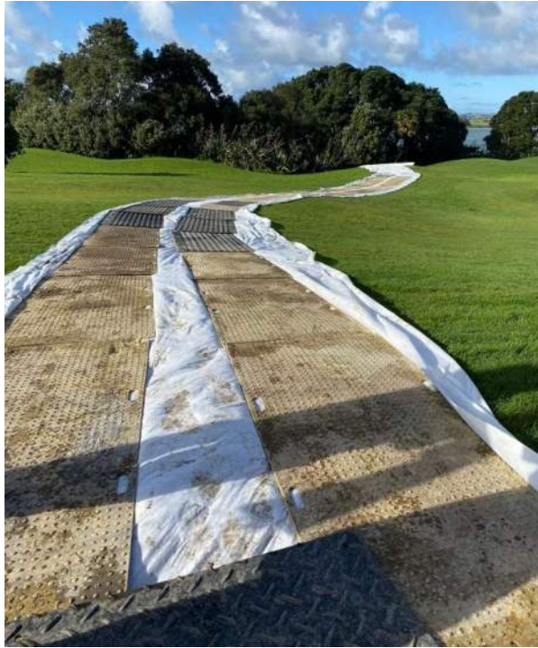
Figure 3: Geotextile and track mats for access tracks
