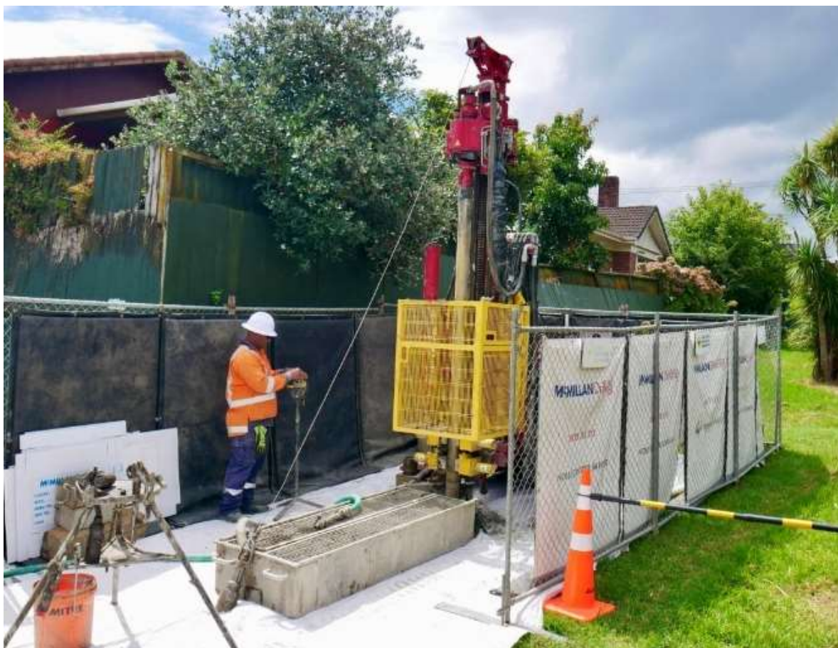
Figure 5: Drill Rig with layout showing temporary fencing, drilling pit and geotextile on ground
