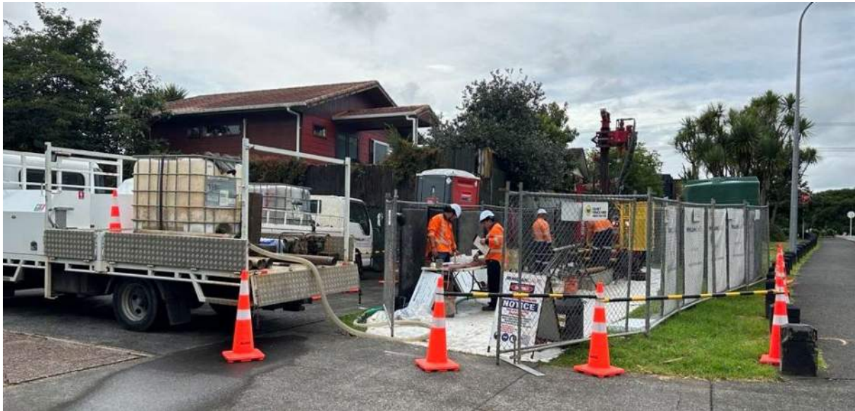
Figure 6: Shows support vehicle, positioning of water tank and engineers in exclusion zone
