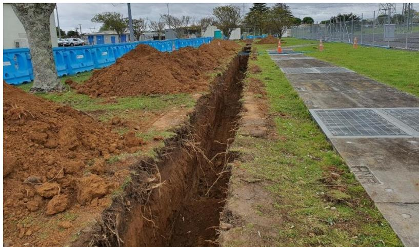
Figure 4-1 Open Cut Pipe Trench
