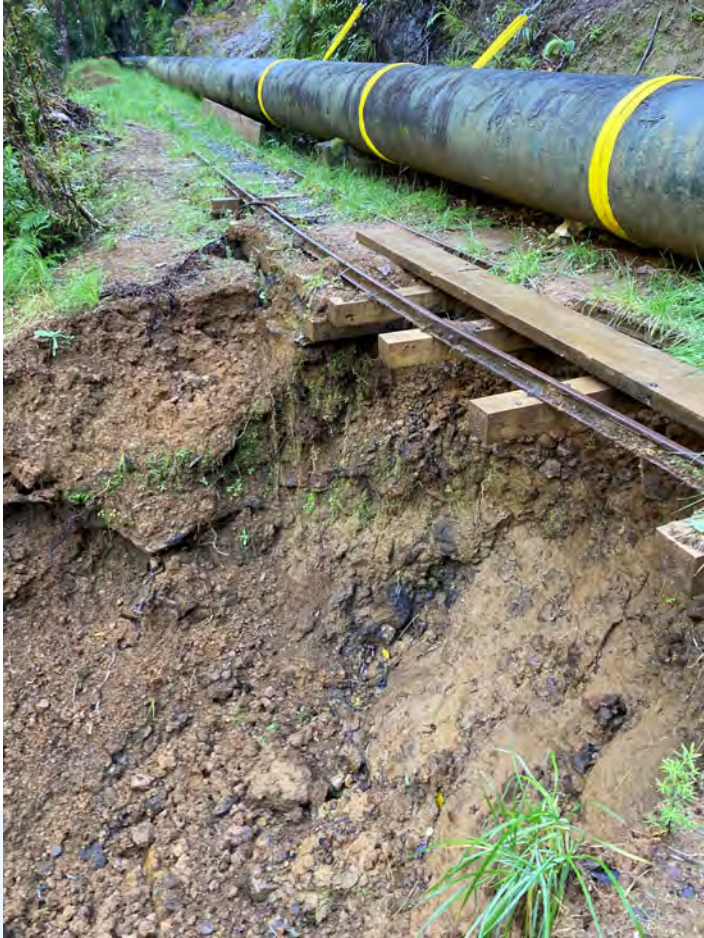
Raw water mains under threat from slips
