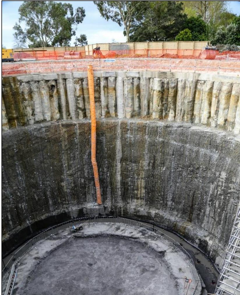
**Figure 3.1 – Shaft Supported by Secant Piles in Soil and Mesh in ECBF Rock**
