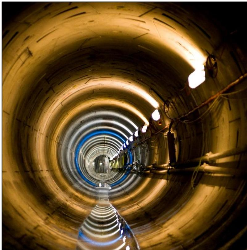
Figure 3.4 – Precast Concrete Segmentally Lined Tunnel
