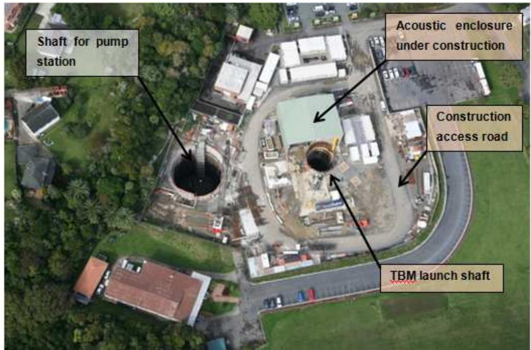
**Figure 8 Typical Primary shaft site appearance (Project Hobson during construction with acoustic shed partially complete to allow 24/7 working in the tunnel)**
