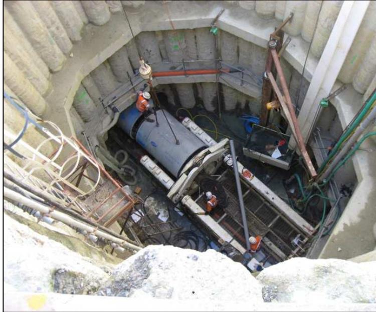
**Figure 5 Set up of pipejacking launch shaft for SW Interceptor**
