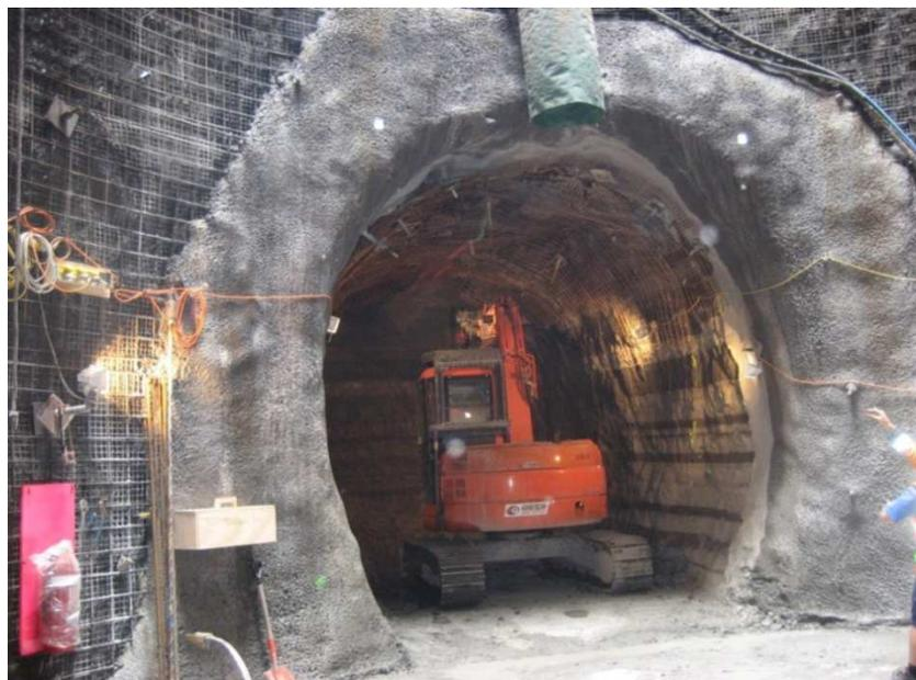
**Figure 7 Typical excavation methods for the de-aeration tunnels. Installation of rock bolts and shotcrete lining are visible (Project Hobson)**
