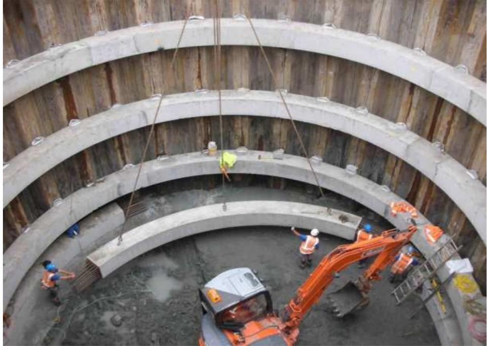
**Figure 12 Typical circular construction shaft in soft ground before excavating down into underlying East Coast Bays Formation rock (Rosedale Project)**
