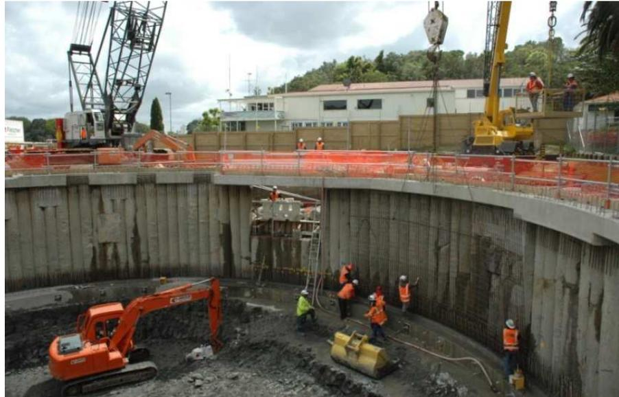
**Figure 15 Construction of the shaft walls for Project Hobson pump station.**
