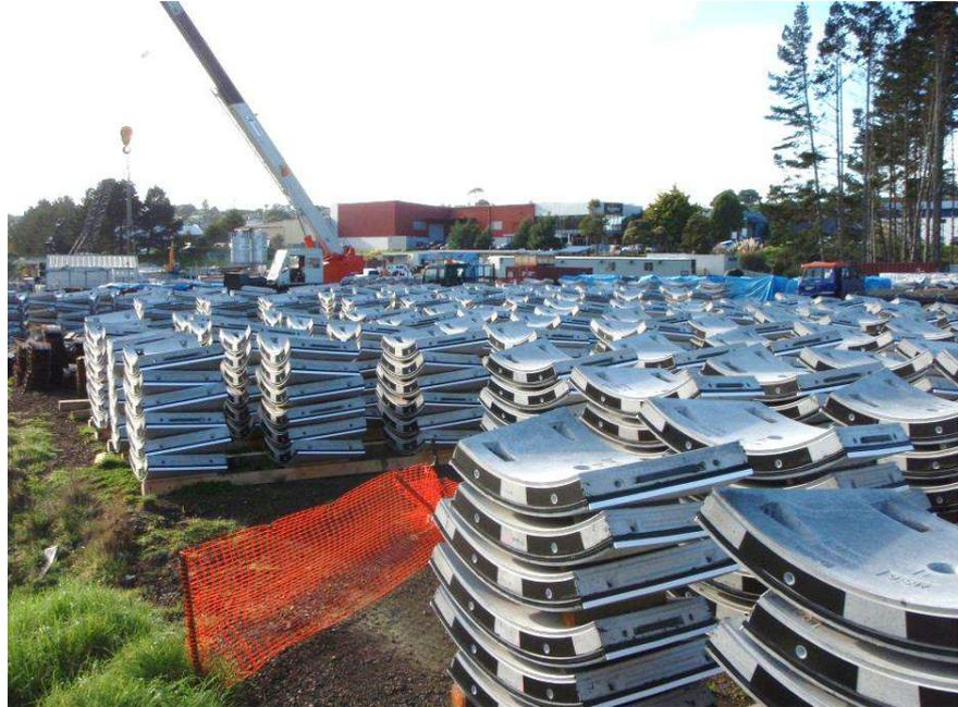
**Figure 3 Tunnel segments being stored ready for use at the Rosedale Project construction shaft.**
