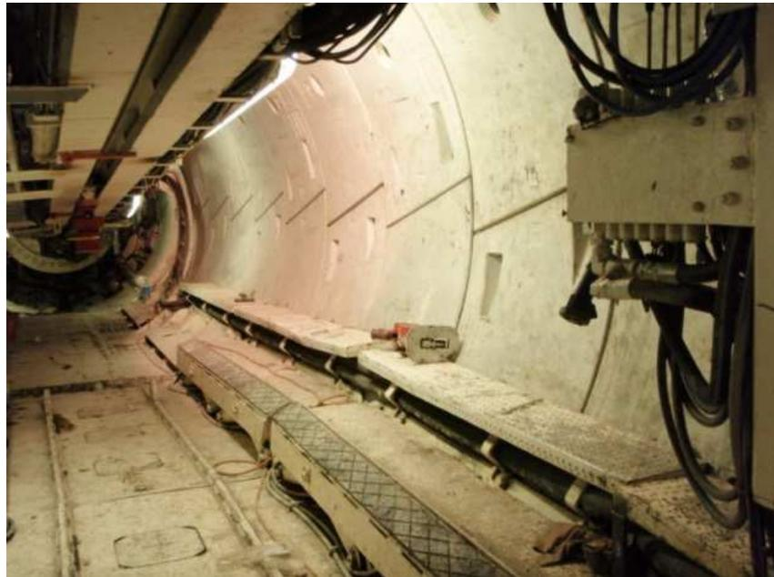
**Figure 2 Typical lining using pre-cast gasketed segments (Rosedale Project)**
