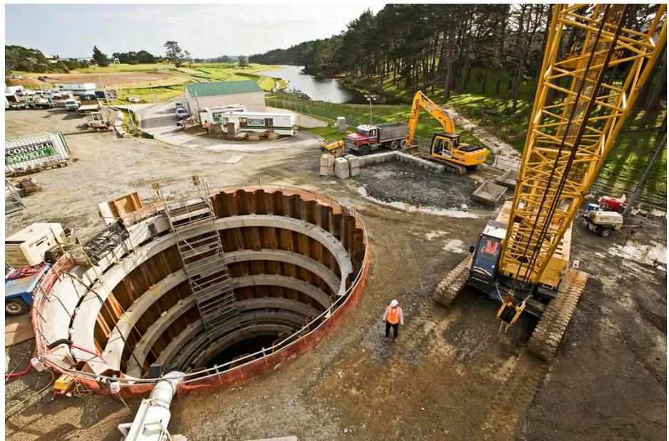
*Figure 2 - Sheet piled shaft excavation during construction for the Rosedale sewer tunnel, source - TunnelTalk.com.*
