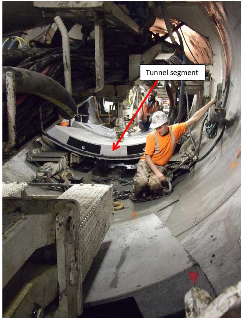
**Photo 1: Precast liner segments being installed on Watercare's Hobson tunnel.**
