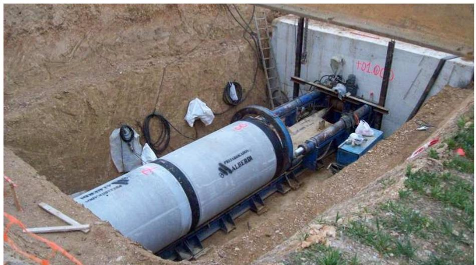
**Photo 2: Precast concrete jacking pipes**
