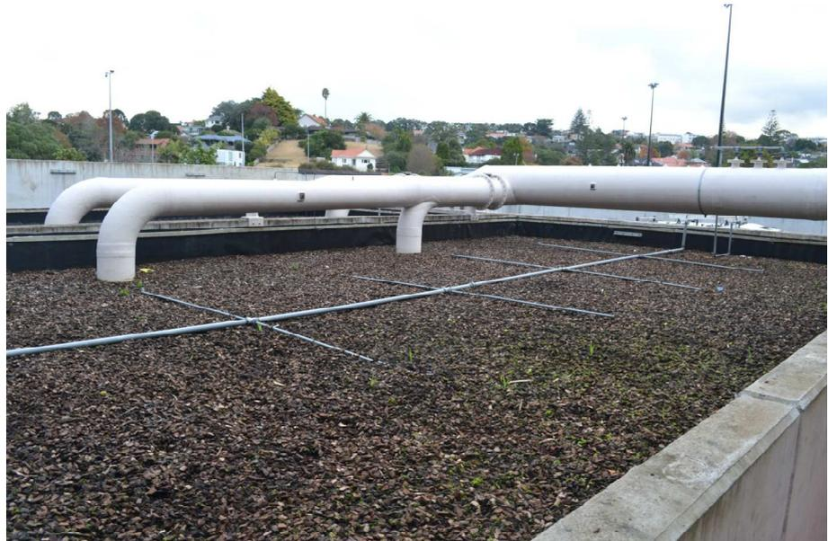
**Photo 3: Bio-filter located at the Project Hobson Pump Station**
