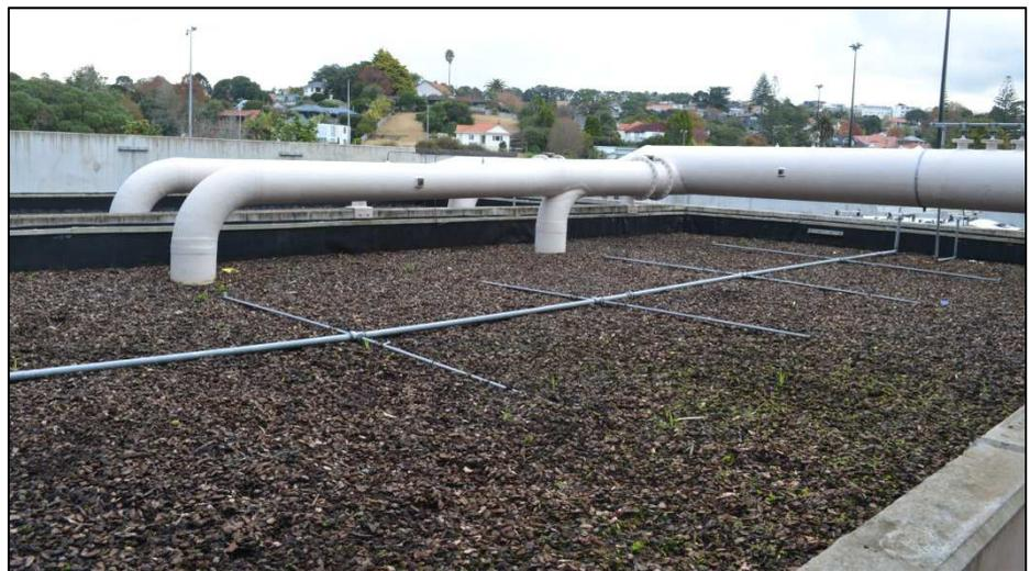
**Figure 1 – Biofilter at Pump Station 64**
