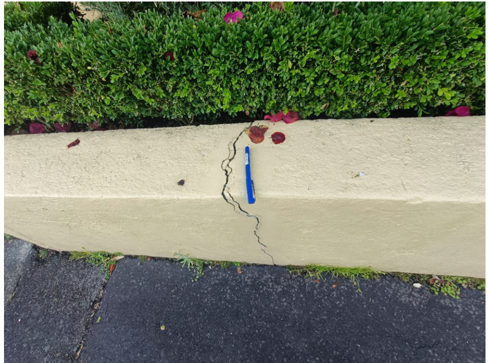
Photo 3 - Example of cracking in landscaping URM walls
