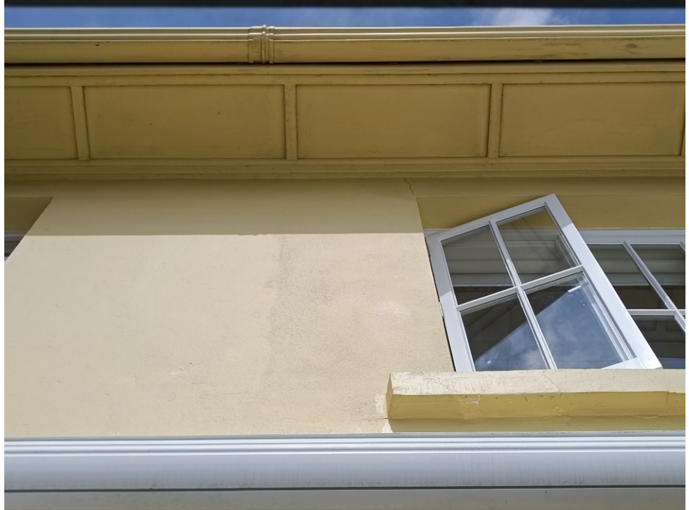
Photo 1 - Example of cracking around windows
