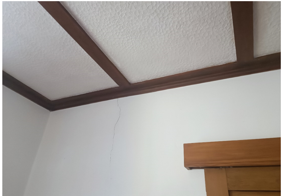
Photo 2 - Example of cracking at interface between URM and timber walls
