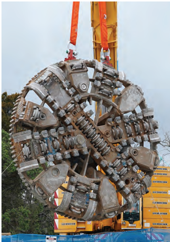
TBM cutterhead being lifted from Pt Erin shaft
