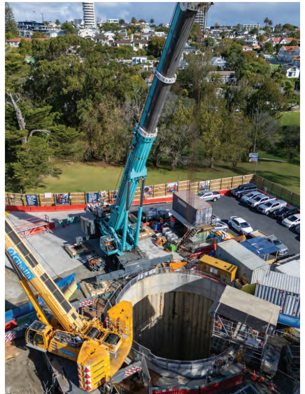
Heavy cranes are needed to remove the tunnel materials
