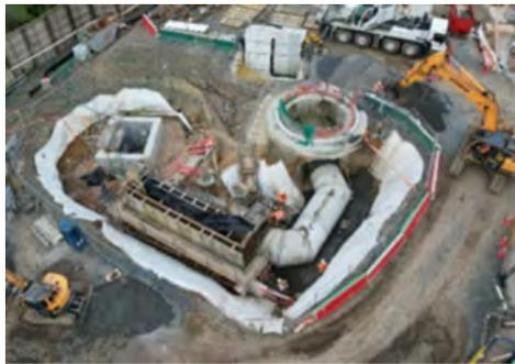
We've now completed all our chambers and are currently installing and testing gates inside some of them. These gates are used to control flow from one chamber to the next. Over the coming months, we will build the remainder of the plant room that will sit above ground level. The plant room will house controls that Watercare operations division uses to operate the wastewater network.
