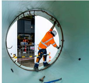
We used a double bracket system in previous drives with brackets every 1.5 metres. Dan came up with an idea to trial a single bracket every 3 metres. This would significantly decrease the number of brackets required and save money and time. This method passed all the necessary tests and Dan’s single bracket system is now the method we apply.
