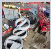
Shaft cascade rings ready for the Mt Albert shaft
