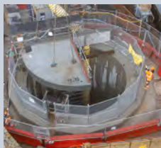
Lowering the cascade shelf into Lyon Ave shaft
