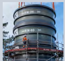
Oversize RPC liners being installed at our Rawalpindi site.
