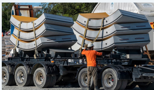
Six segments for just one ring makes a big load - Mar 2023
