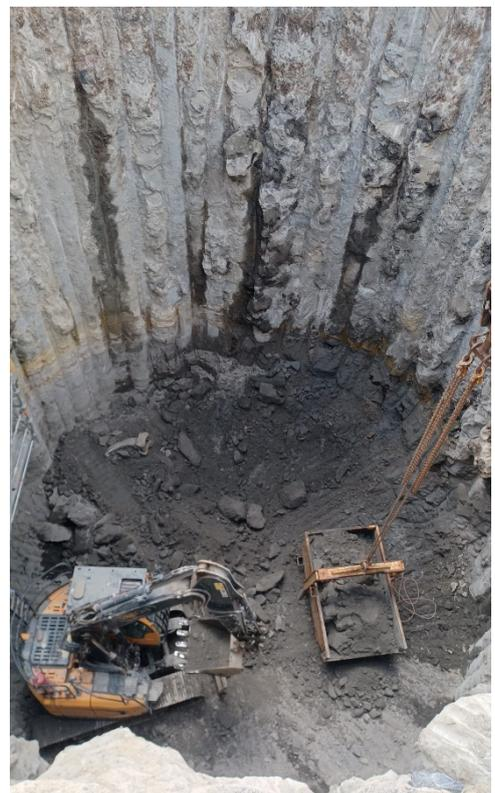
Figure 6 Typical Secant Pile shaft under Excavation
