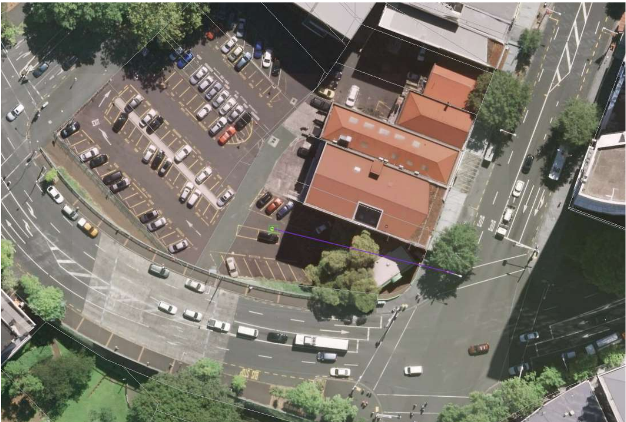
Figure 3-1: P3-P4 connector tunnel existing environment
