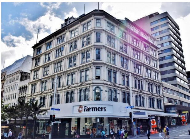
Figure 4: The former John Courts Building, now known as the Farmers Building.
