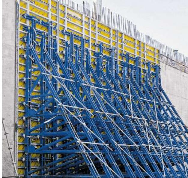
*Figure 10 - Example of single-sided formwork system*
