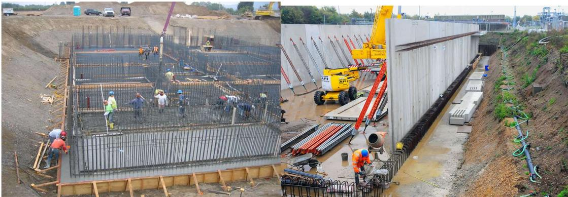
*Figure 6 - Example typical slab and cast insitu wall construction (left) and pre-cast panel (right)*
