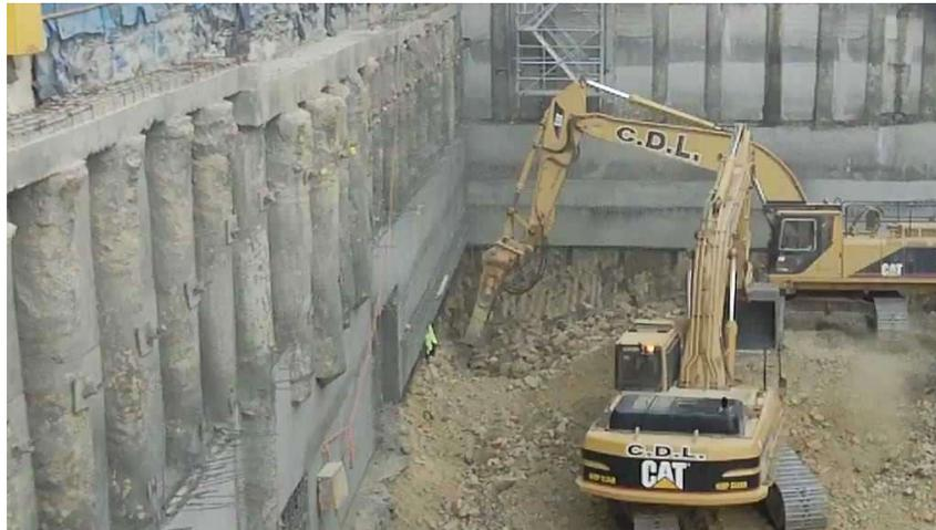
*Figure 9 - Example Ground Retention and Bulk Excavation*
