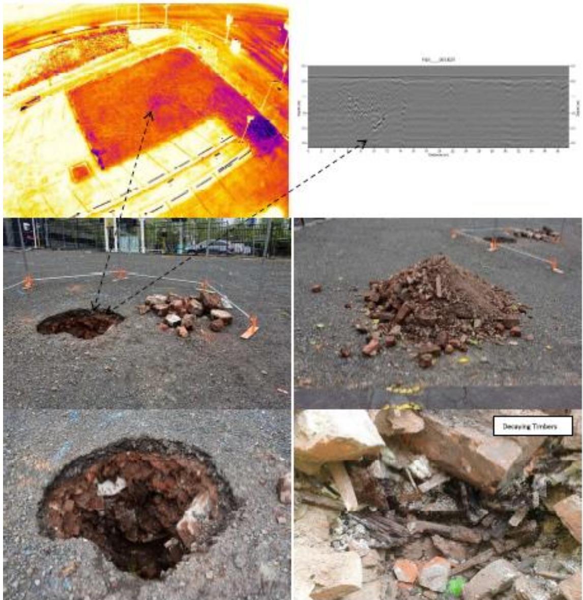
Figure 18. Showing pothole excavation (PV1) undertaken by Briton Detection and Inspection in the Greys Avenue carpark in 2019, exposing building demolition rubble (Eggleton 2019)
