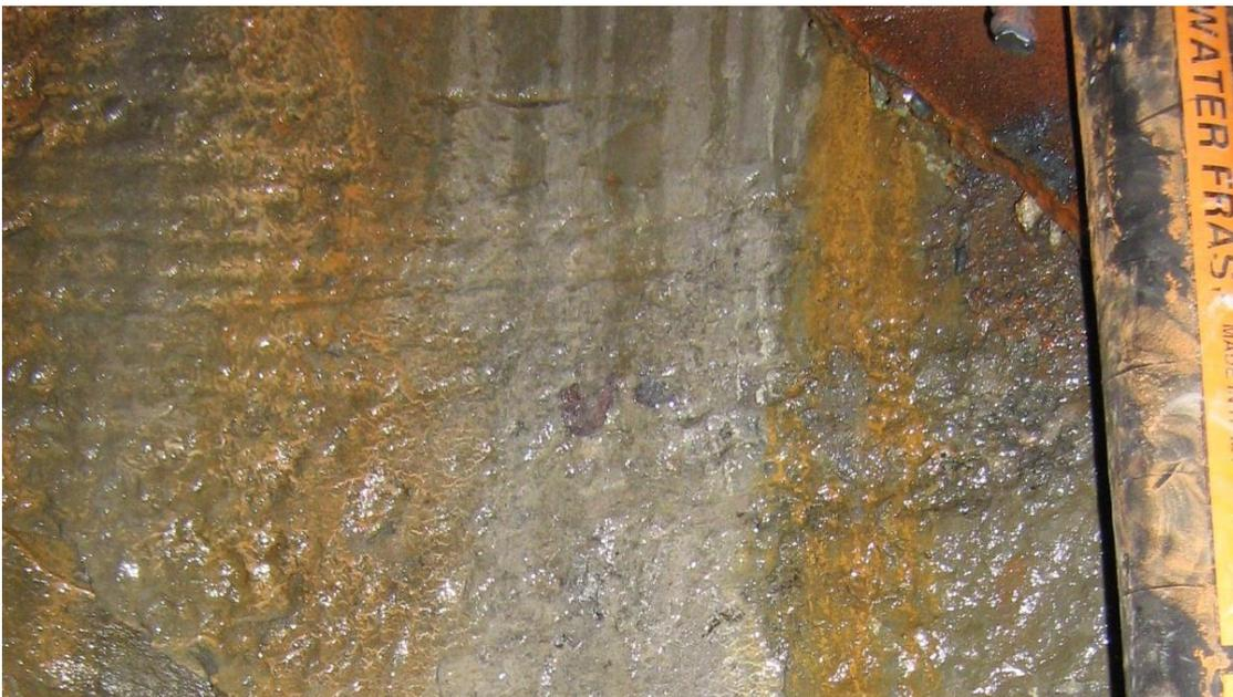
Figure 3.4 : PVC in the face of the Davis Crescent tunnel. This rock was well cemented with calcite and recorded a uniaxial compressive strength in the order of 10-20 MPa. The largest grain (dark red grain near photo centre) is 14 mm across.
