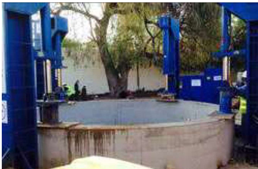
Figure 4 Typical photo of jacked caisson shaft sinking method
