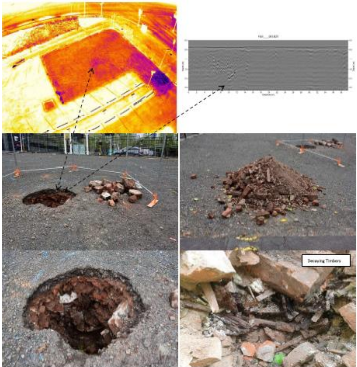
Figure 16. Showing pothole excavation (PV1) undertaken by Briton Detection and Inspection in the Greys Avenue carpark in 2019, exposing building demolition rubble (Eggleton 2019)
