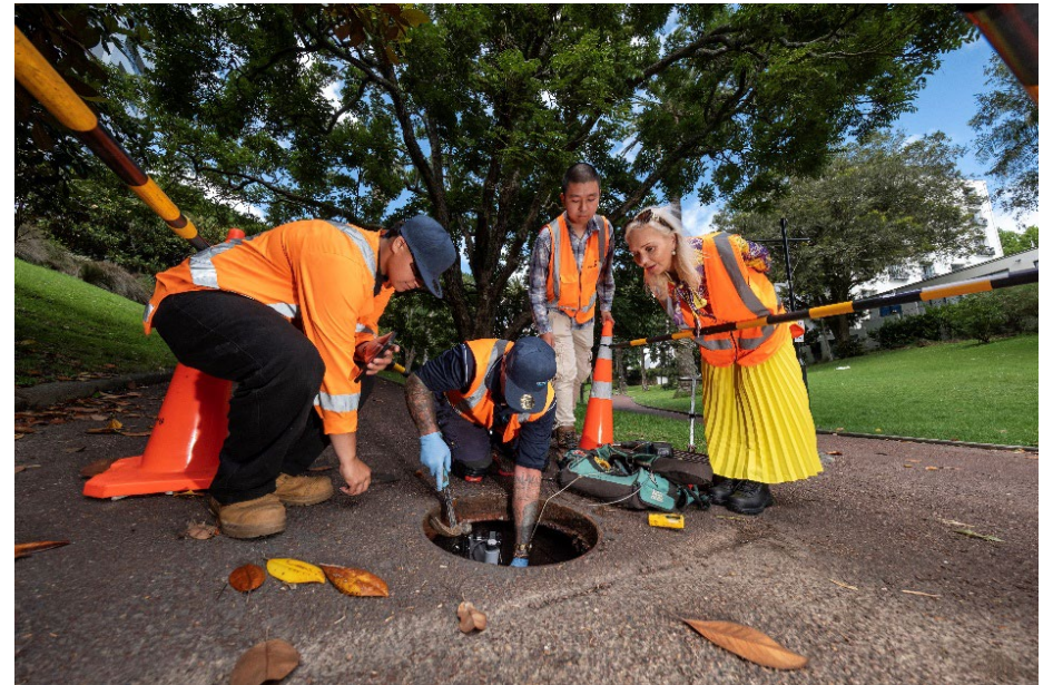
Deputy Mayor Desley Simpson visited Myers Park where we are installing smart sensors into the wastewater network, which give us daily insights into what is happening in the pipes below ground so we can better predict and prevent blockages.
