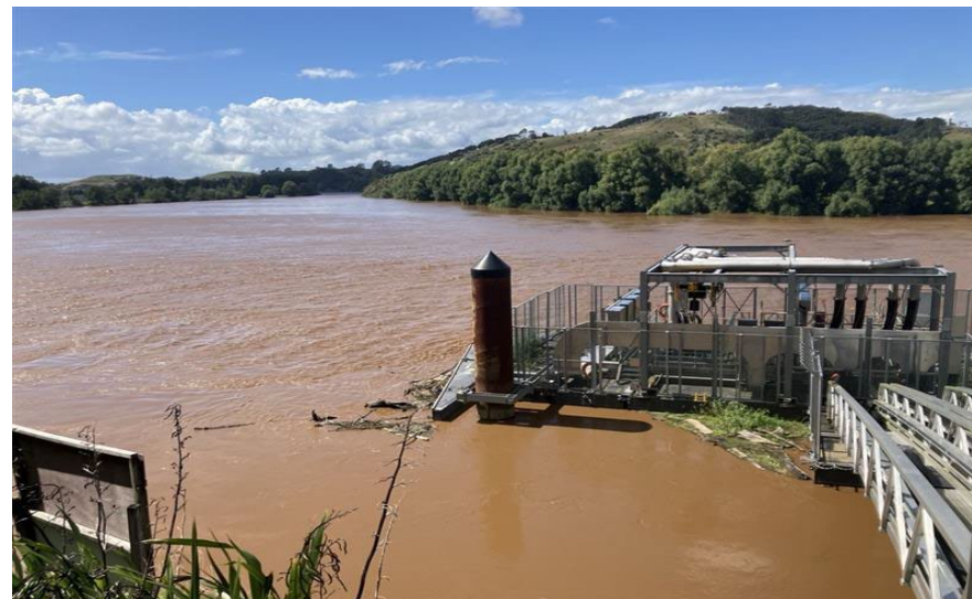
Waikato water treatment plant after severe flooding event in February 2026
