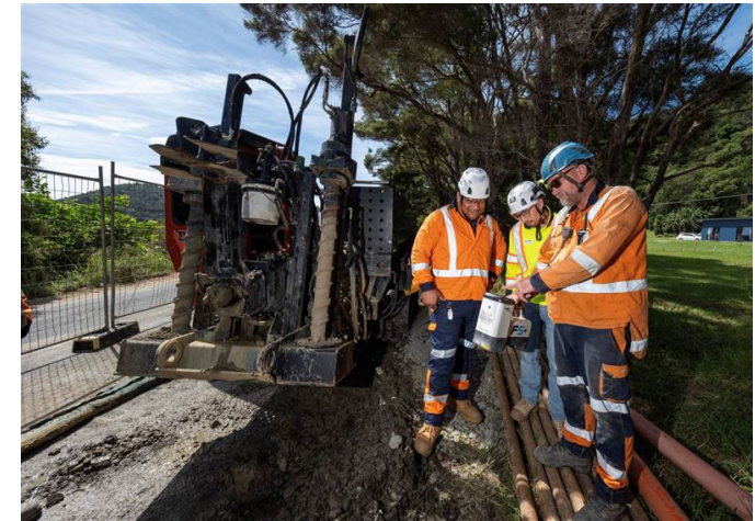
Crews work to install a 4.5km wastewater main that will transfer wastewater from Waiwera to Hatfields Beach pump station.
