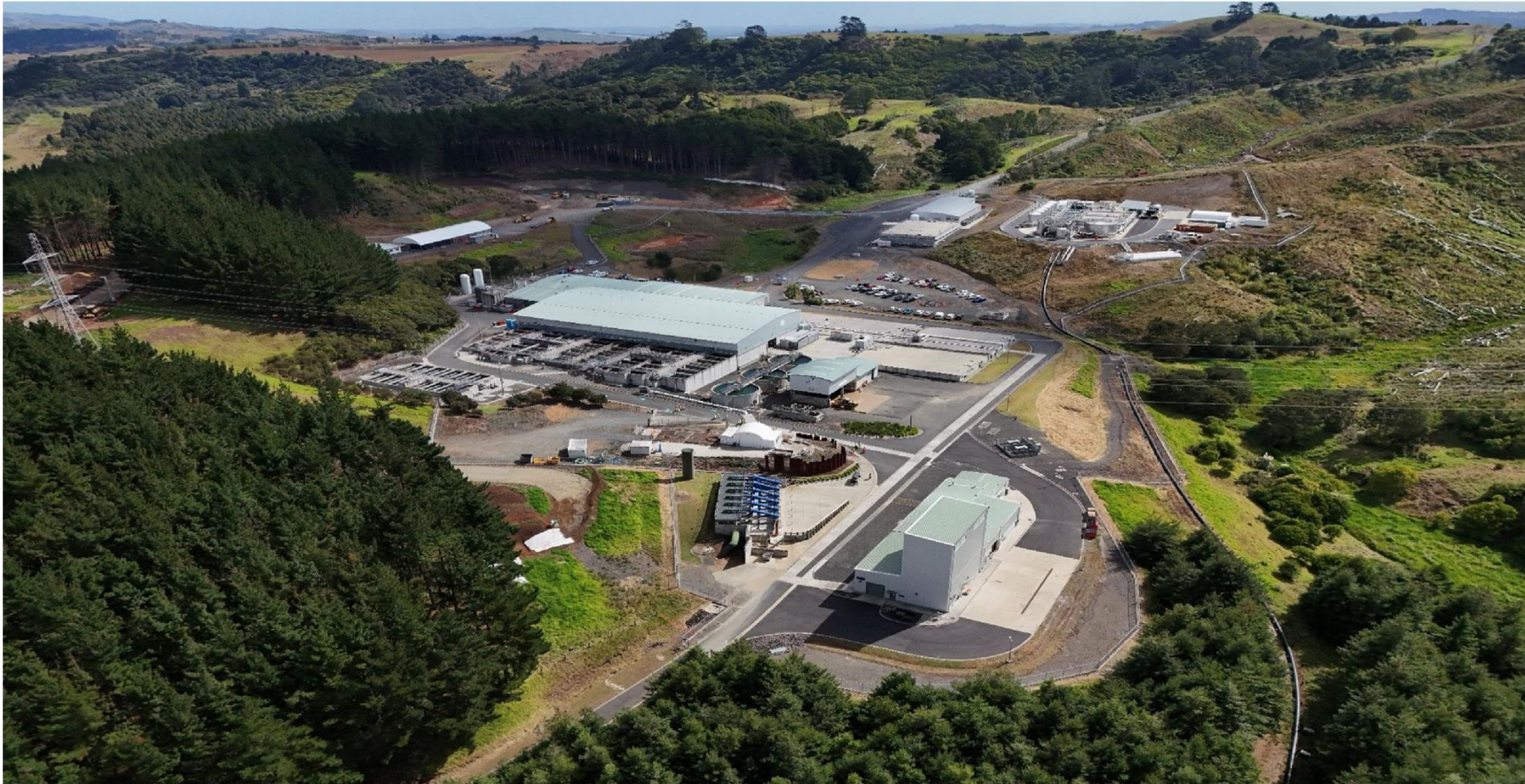
Waikato Water Treatment Plant in Tuakau
