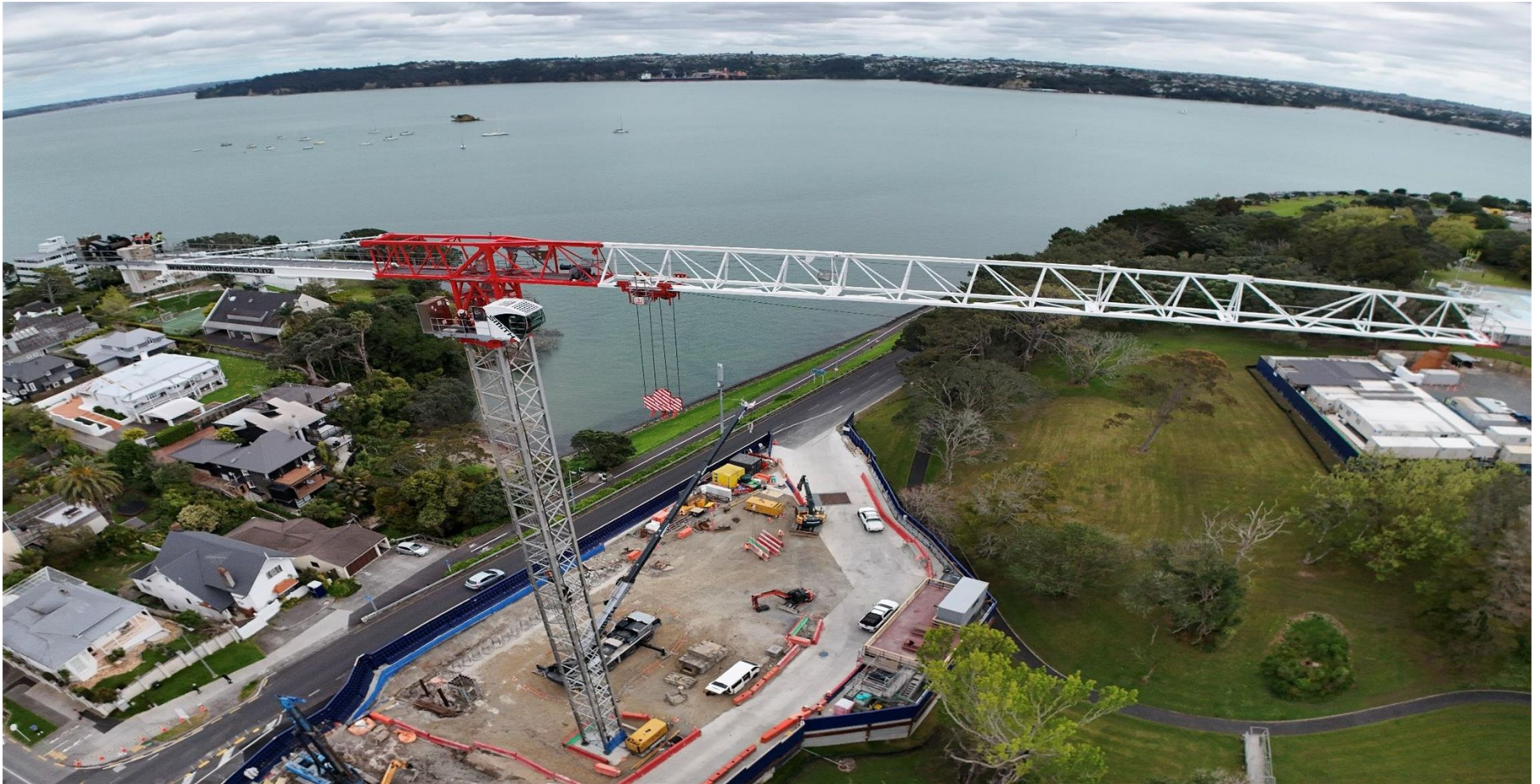
The tower crane that has been set up to build a control chamber that will divert flows from the Herne Bay Collector into the Central Interceptor
