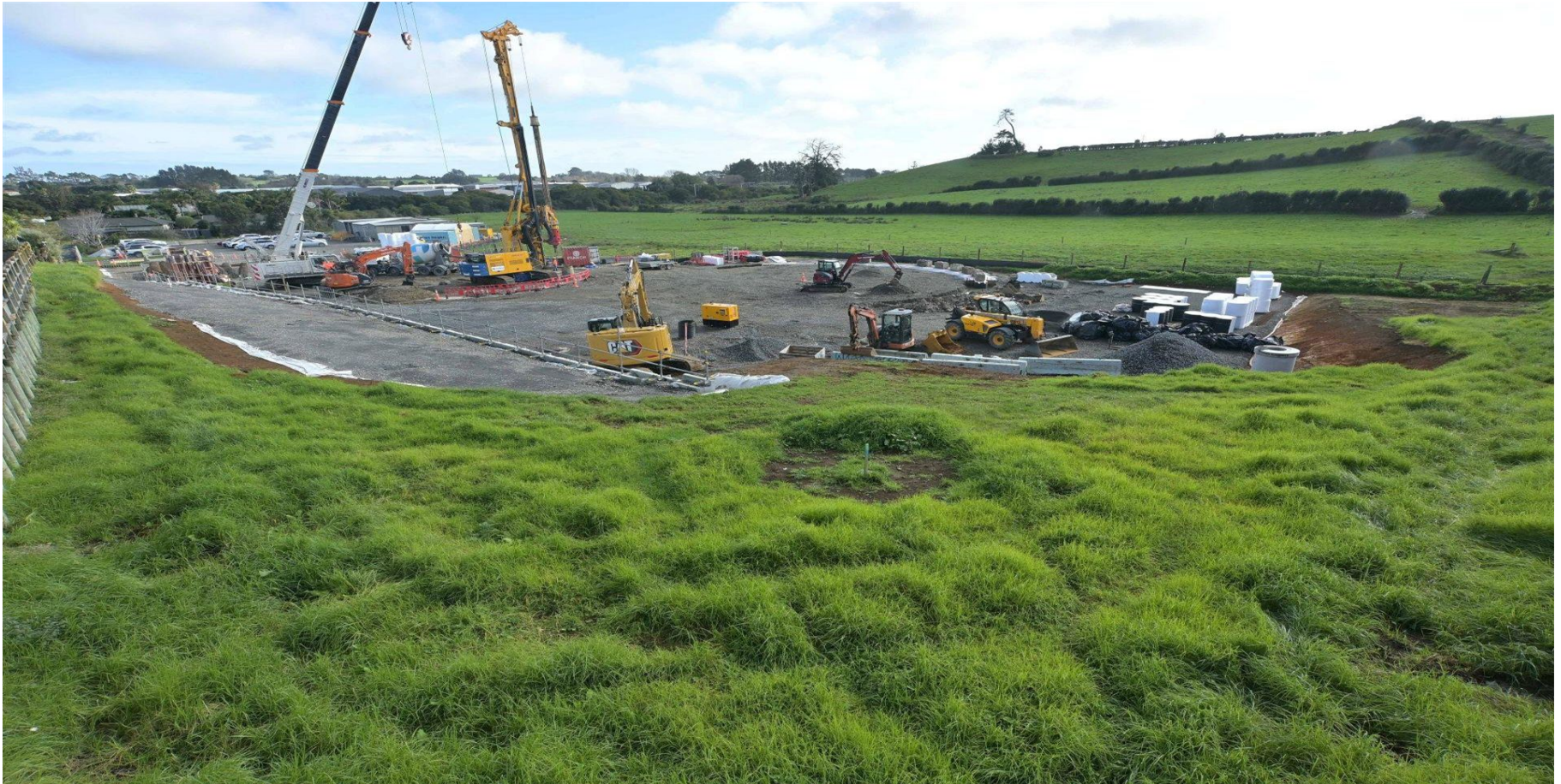
Early works underway on the new wastewater pump station on Isabella Drive
