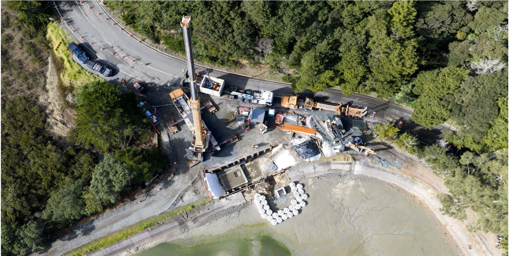
Aerial view of the Waiwera Pump Station installation
