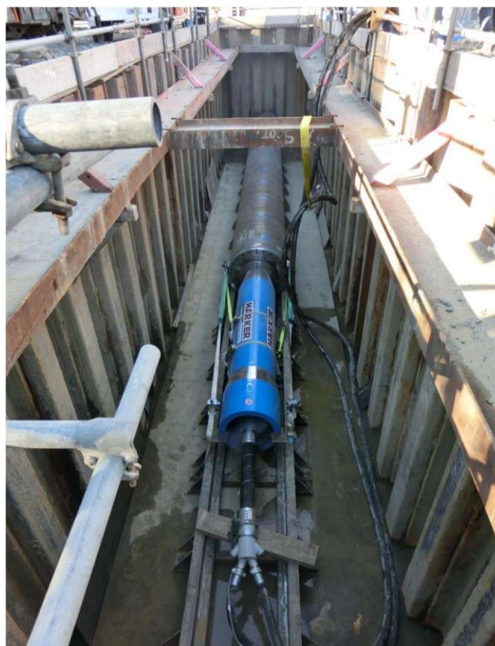
Figure 22. Photograph of indicative pipe hammering set up (Source: Brian Perry Civil)
