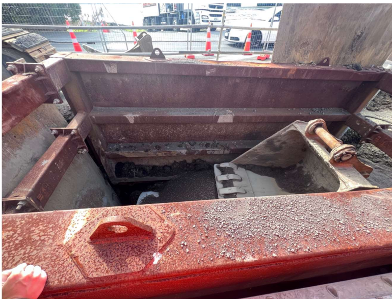
Figure 21. Example of open trenching using trench shields (Photograph: Tingran Duan, 2 September 2022)
