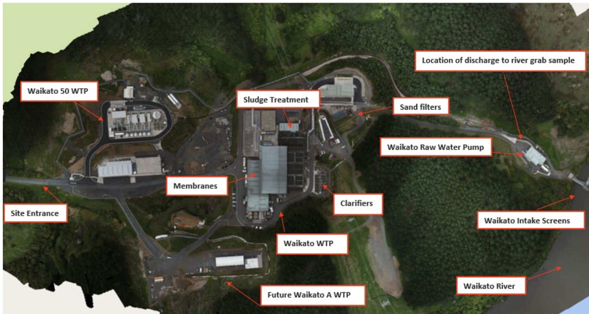
Figure 2-1: Waikato WTP site overview
