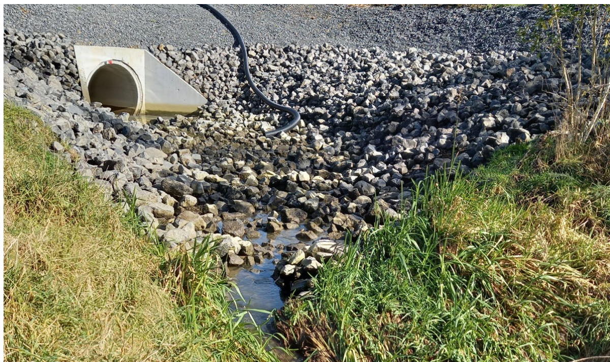
Figure 4-11: Discharge outlet location into the Wairiri Stream. View looking upstream.
