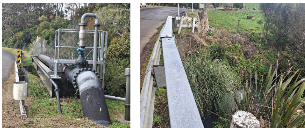
Figure 4-8. The Parker Lane pipe bridge.
