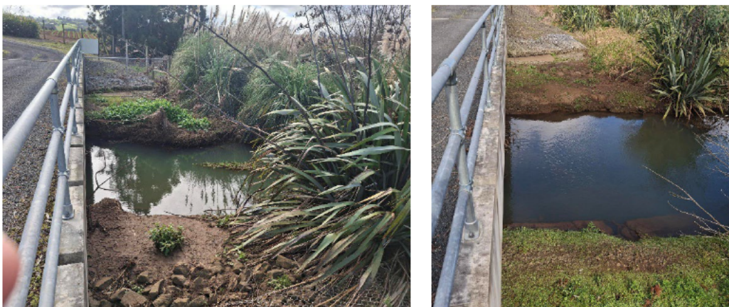
Figure 4-10. The channel under the vehicle bridge
