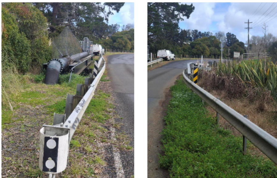
Figure 4-9. The treatment plant entrance pipe bridge.
