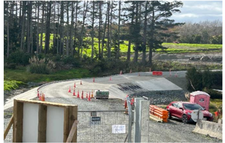
New Culvert and Ford on Hamatana Access Road
