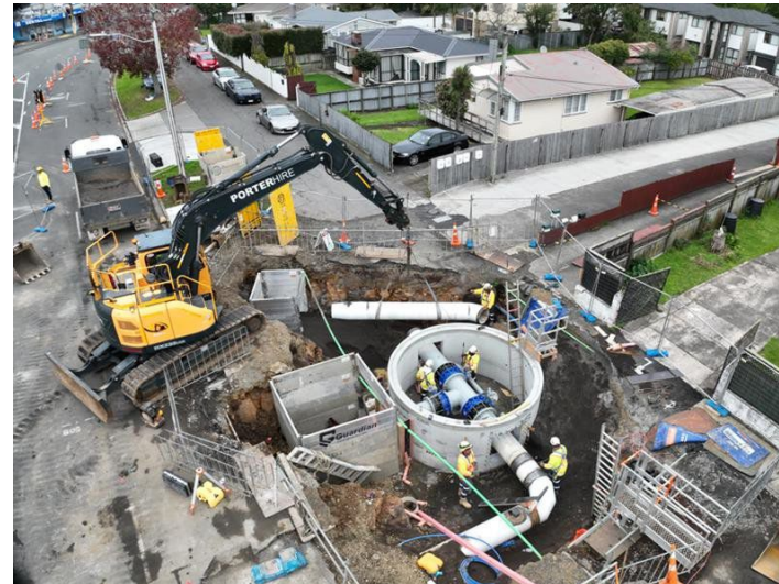
O'Donnell Road – Valve Chamber
