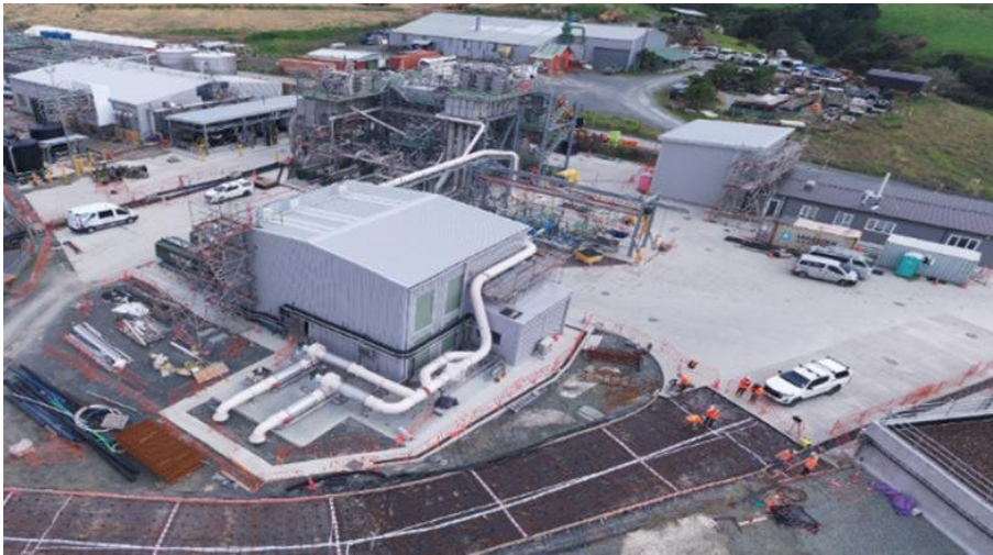
Dewatering building with new access and odour pipework
