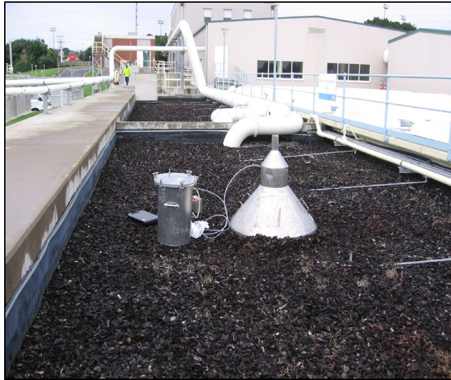
Figure 13: Sampling the Screening Building biofilter (zone 2)
