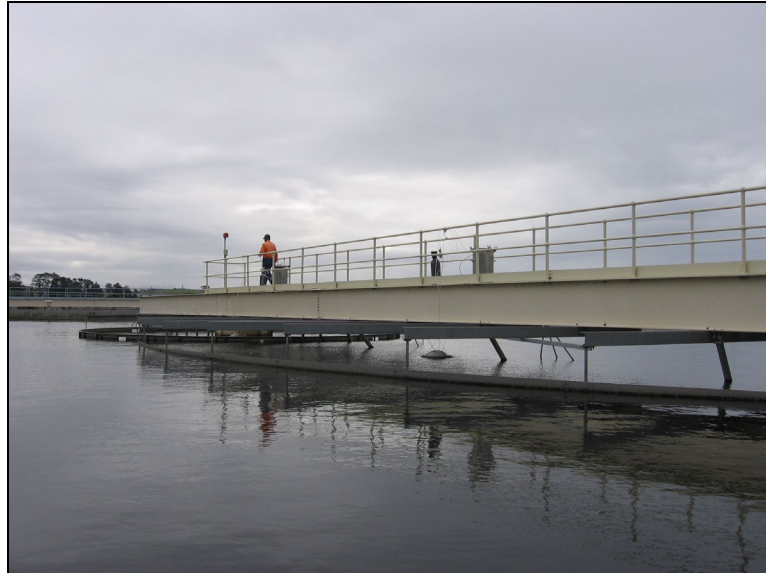
Figure 9: Inner zone and outer zone sampling on a clarifier
