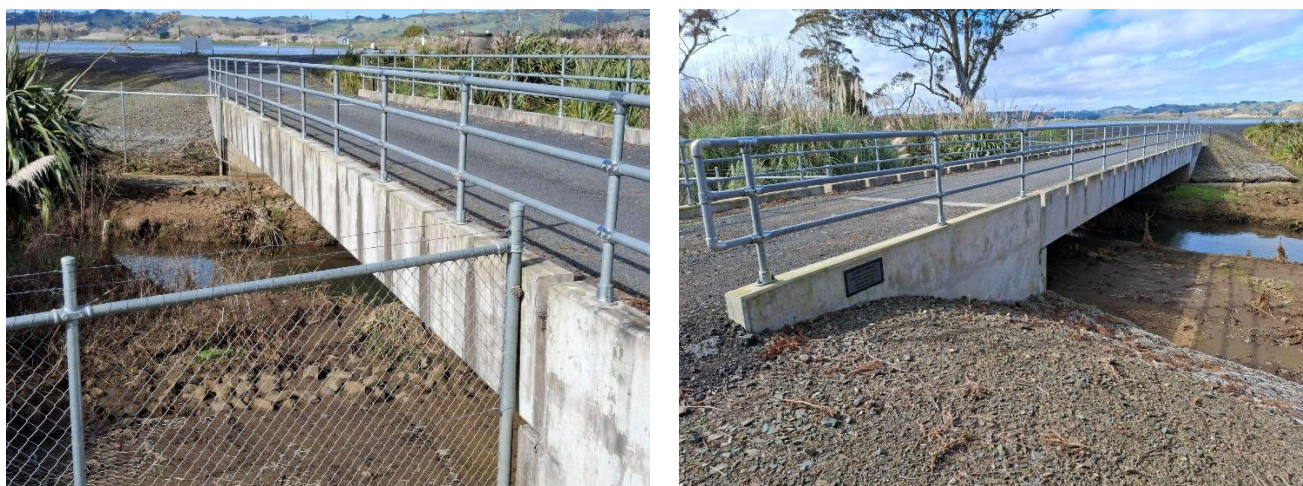
Figure 3-3 The channel under the vehicle bridge
