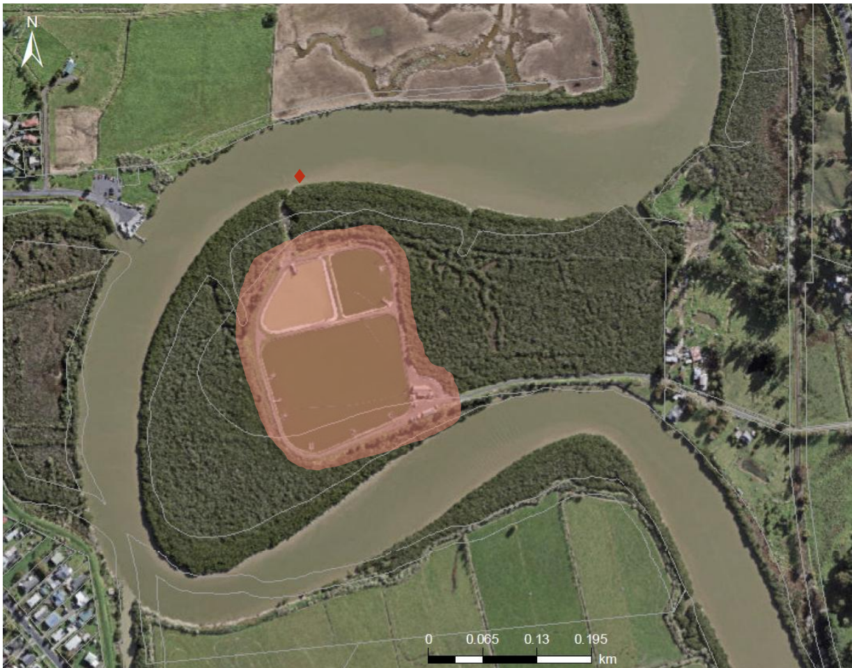
Figure 2-1 Aerial image of the Helensville WWTP (highlighted red) with location of discharge point (red diamond)
