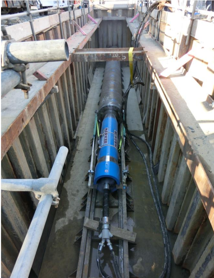
Figure 9 – Indicative pipe hammering set up.
