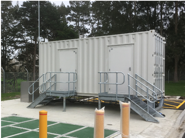
TYPICAL CONTAINER INSTALLATION FOR A PUMP STATION
