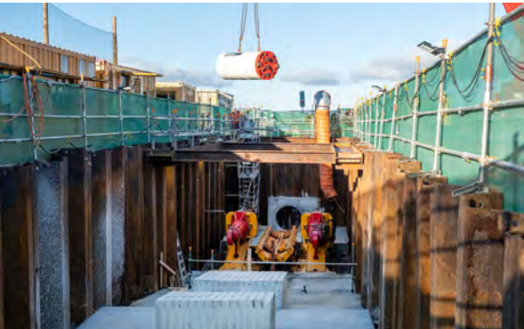
The tunnel boring machine is lowered into the launch site by crane.
