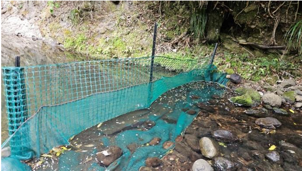
Plate 1 – Temporary fish barrier installed at Site B – Waitākere River. 4 March 2025.
