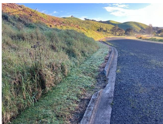
C: Swale 3, looking downhill towards front gate
