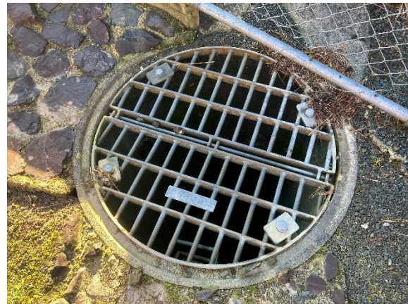
B: Drain and grate from southern aspect of the western swale
