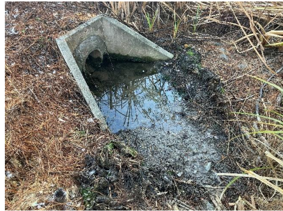
B: Southern aspect of western swale outlet
