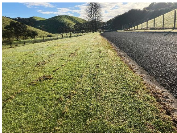
A: Swale 1, looking downhill towards front gate
