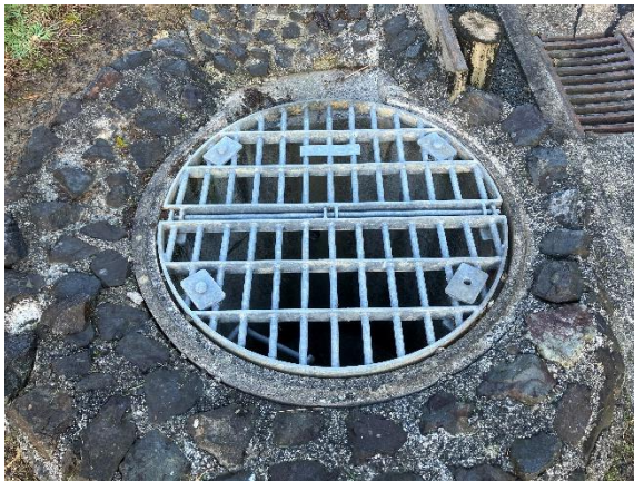
A: Drain and gate from northern aspect of western swale
