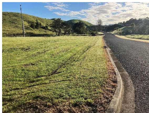
B: Swale 2, looking downhill towards front gate
