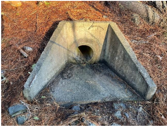
A: Stormwater 360 cartridge outlet
