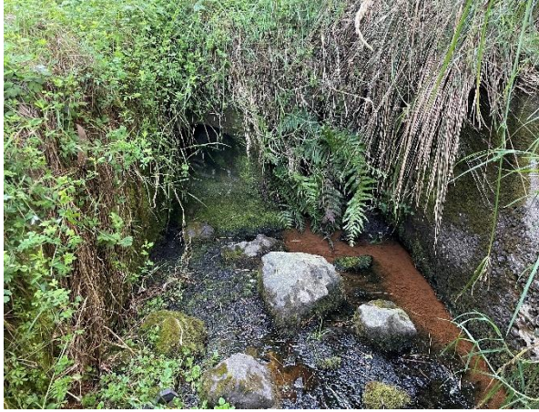
a) Outfall structure (left)
