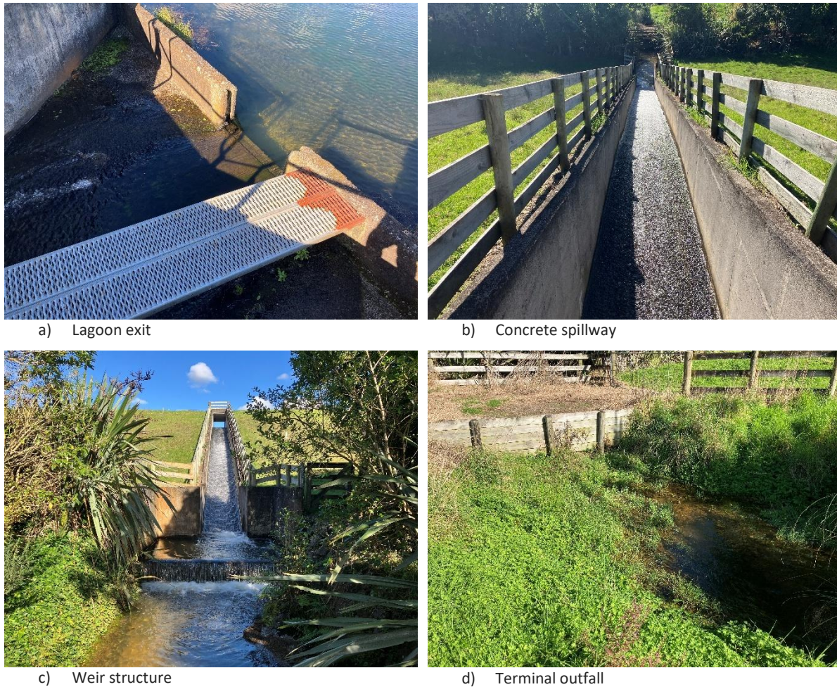
Figure 9: Outfall structure 1 photos.
